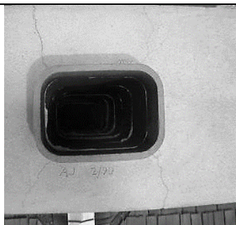
Clay Tile Liner Flue
