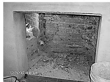
Badly Deteriorated Firebox
